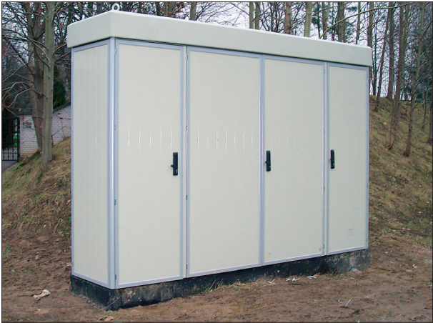
The cabinet after extension
