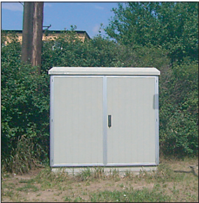
Cabinet before extension
