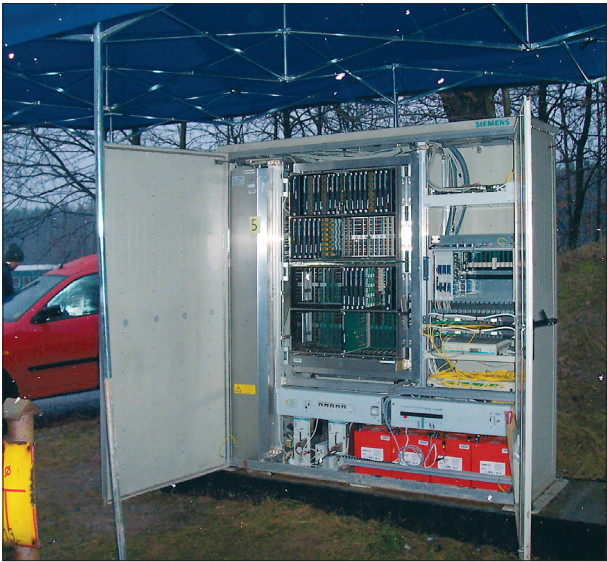
Cabinet before extension
