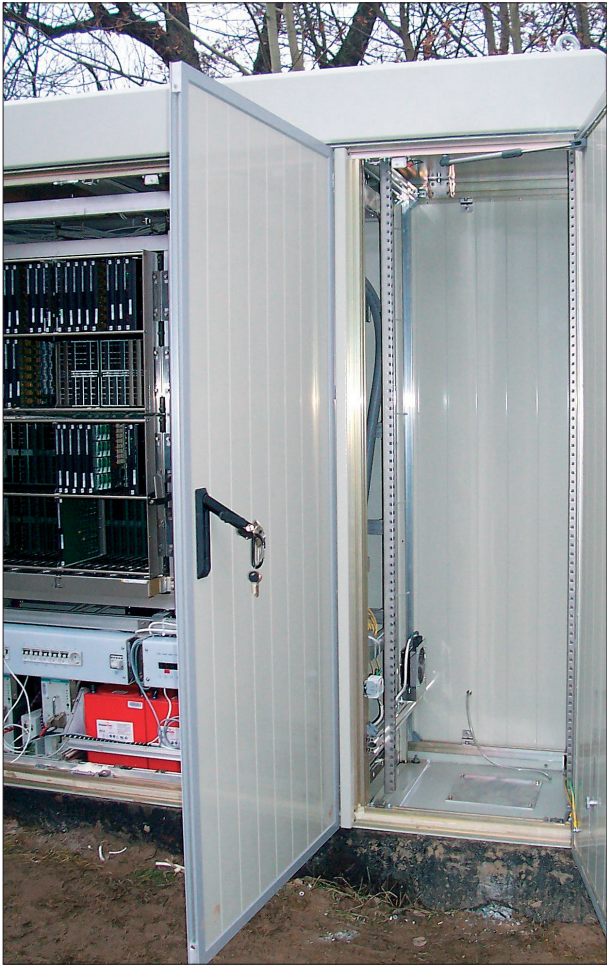
The cabinet after extension
