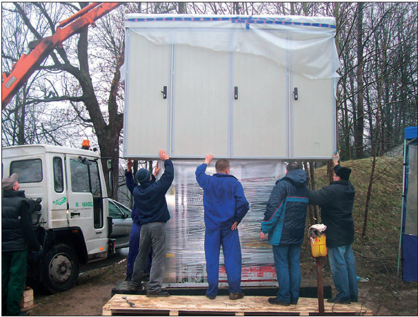
Cabinet during extension
